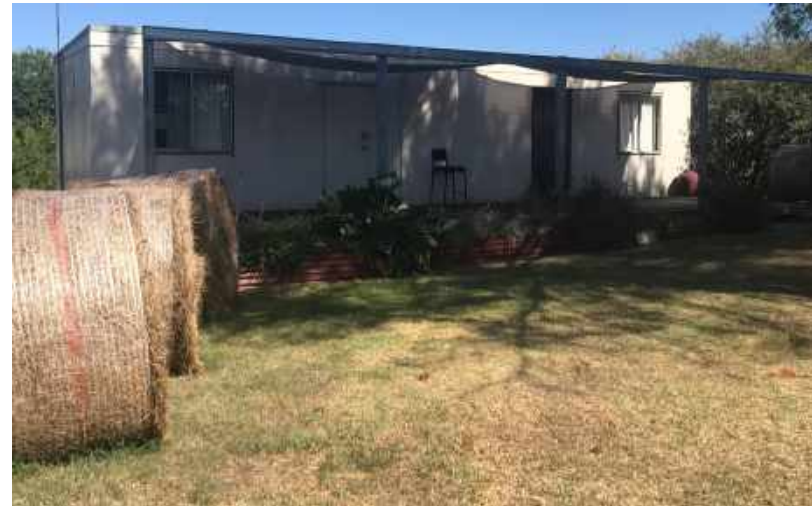
Figure 3.4.14 Donga Building B (left) and Donga Building C (right)
